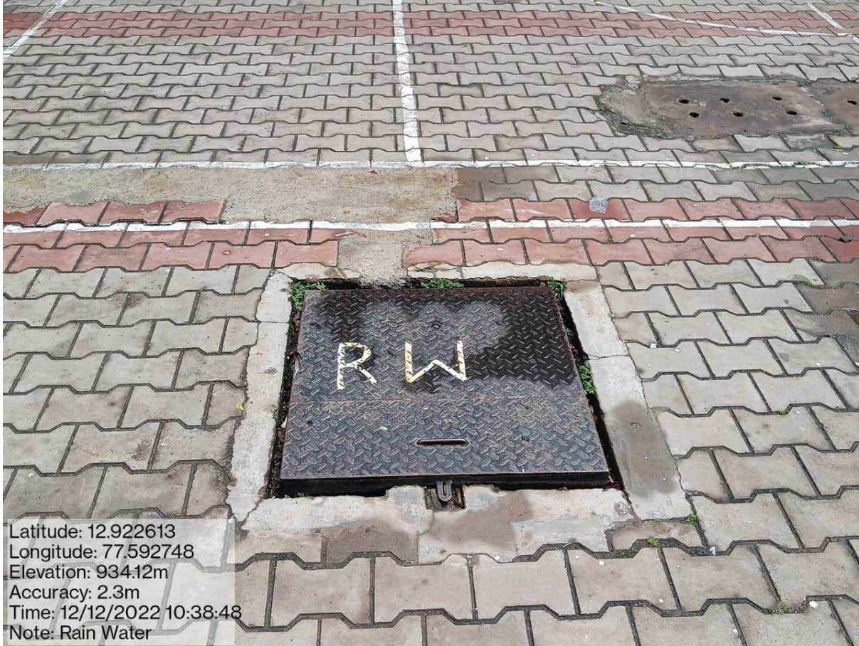
Rainwater Collection pit in the Campus
