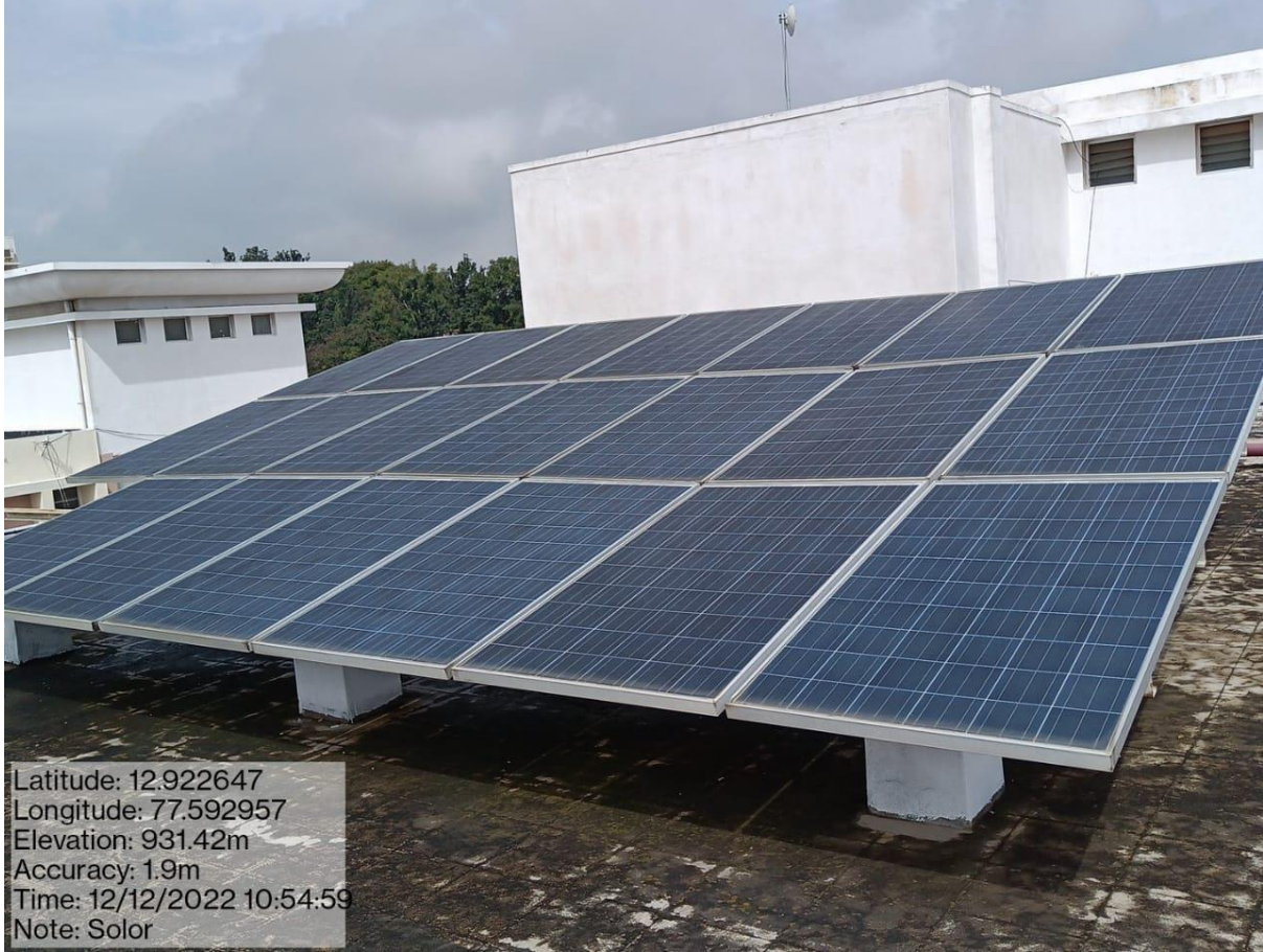
Solar Panel installation on the campus
