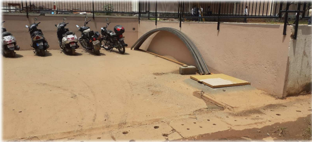
Underground water storage tank
