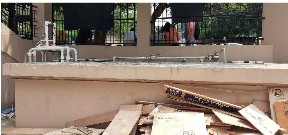
Underground water storage tank
