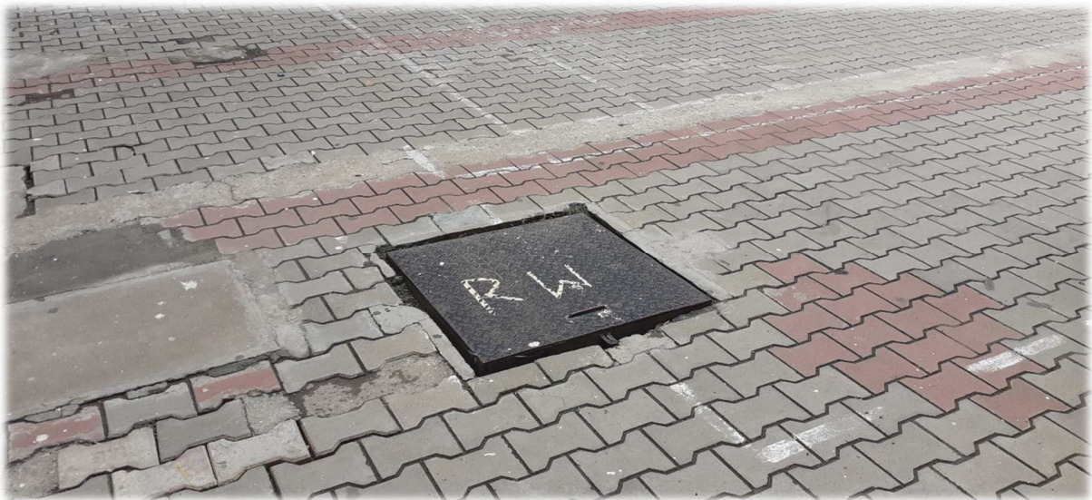
Underground water storage tank for Rainwater
