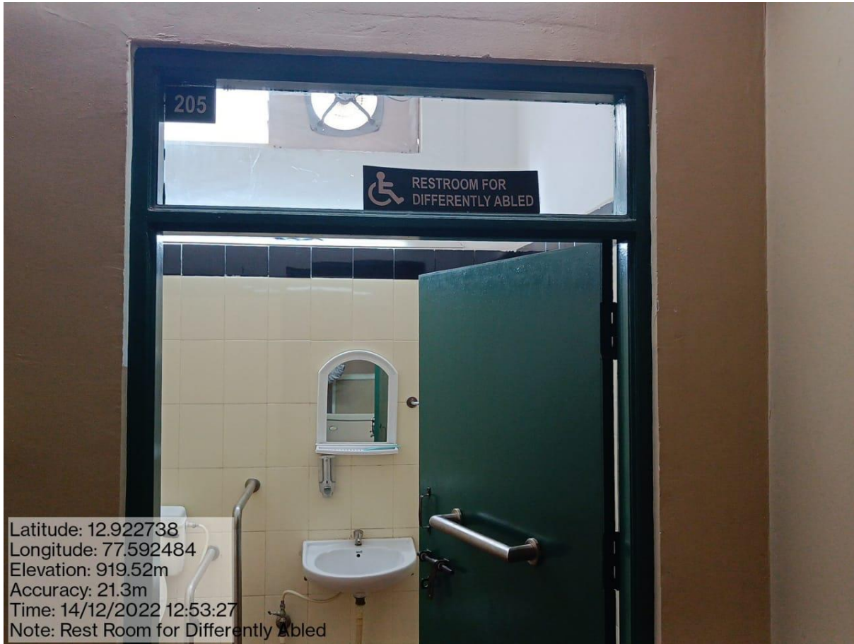
Separate Washrooms earmarked for Differently -abled.
