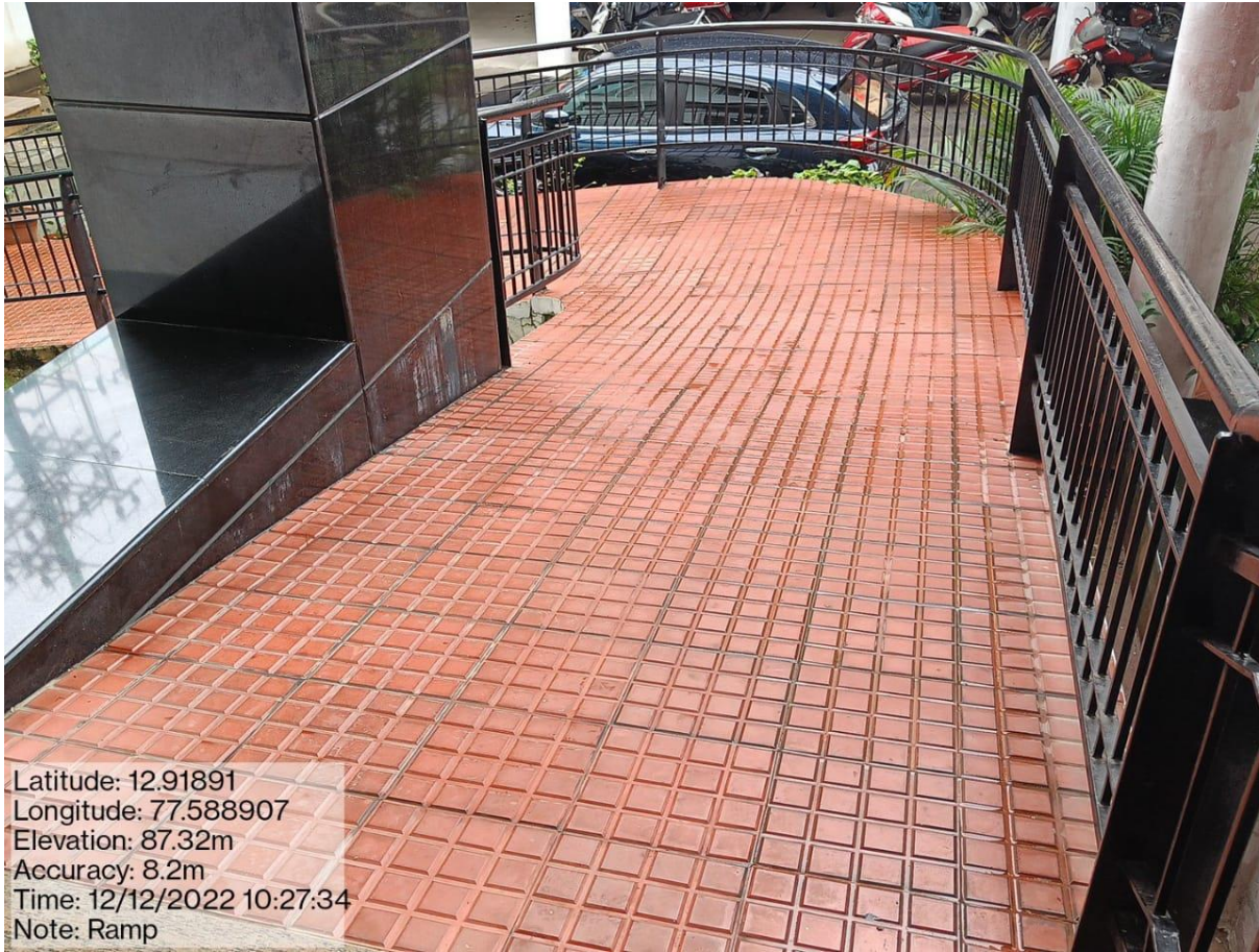
Ramp in the college entrance for easy access to the differently-abled.
