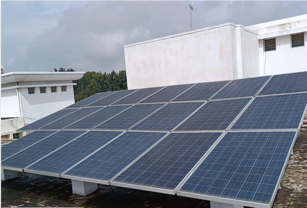
Solar Panel installation on the campus
