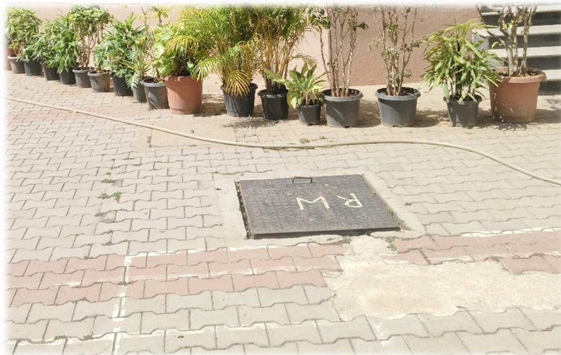
Rainwater storage tank
